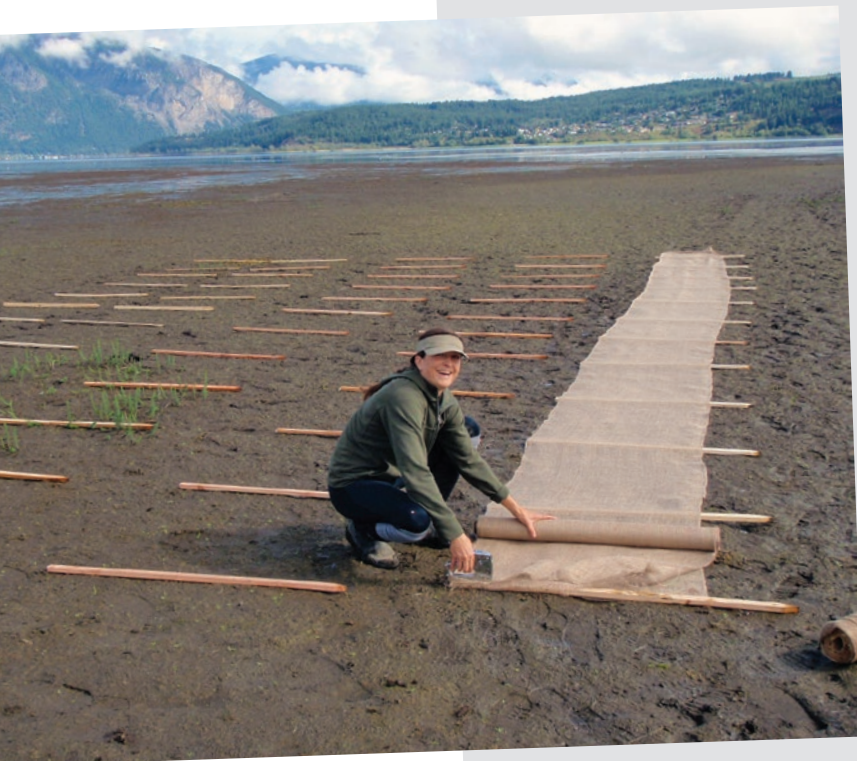
Tracy building silt fences to help get Chinook up the Salmon River
