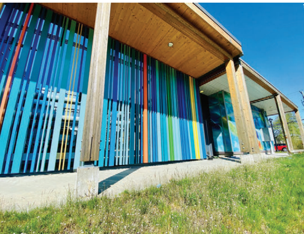
1 A view of the multi-award-winning Alexandra District Energy Utility in Richmond, BC
