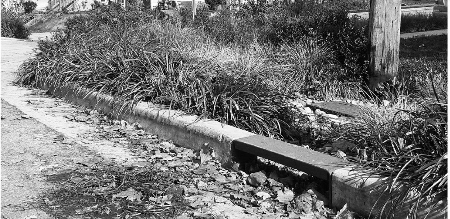
Perforated curbs reduce effective impervious areas by allowing runoff from the street to infiltrate and evaporate in a rain garden instead of flowing into the stormwater pipes at Clark Park in Vancouver's Kensington-Cedar Cottage. Credit: Camille Lefrancois
